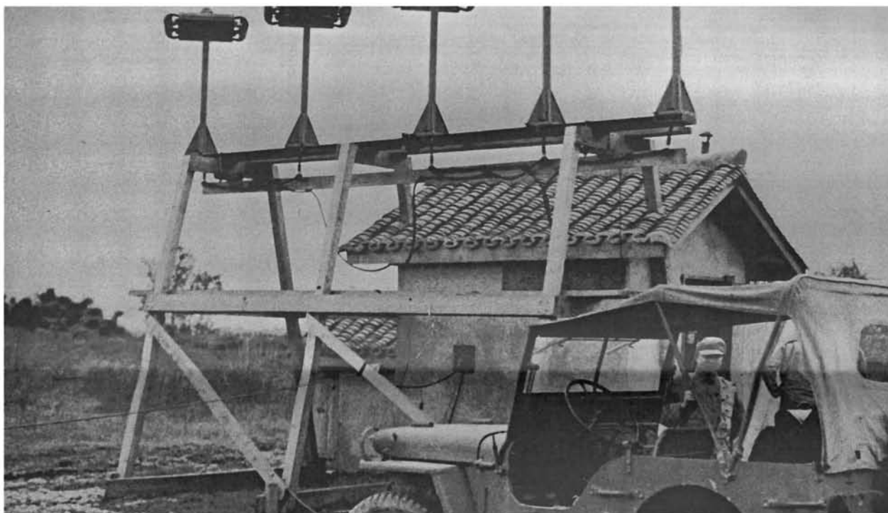
This was a localizer glide-path radar unit used by the 4th Army Airways Communications System Wing based at Kuang-han Air Base (northeast of Chengtu). The picture was taken in November 1944.
