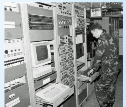
A1C Mark Williams checks the status of Digital European Backbone remote unmanned sites using transmission monitoring and control equipment, Europe.
