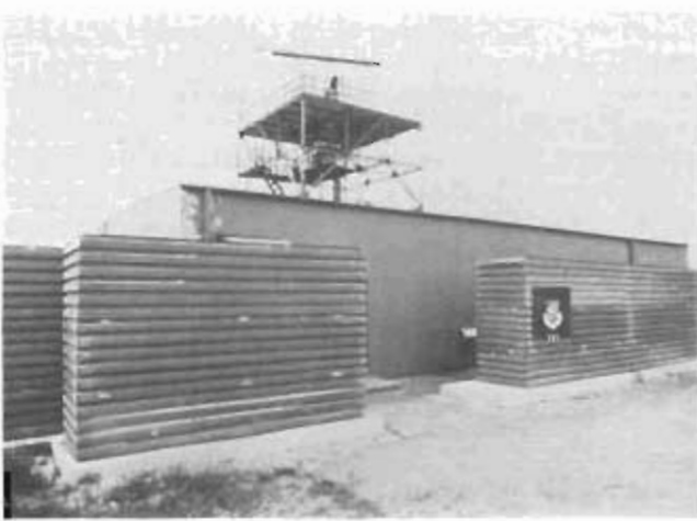
Revetments, such as these at Aviano AB, Italy, were designed to give AFCC sites added protection from attack.
