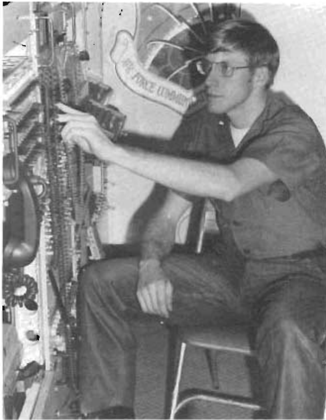
An AFCS officer adjusts controls on a transportable technical control facility employed as part of the Defense Communications System contingency station. The technical control center is a semi-trailer van containing equipment that provides voice and teletype circuits and signal patching and monitoring.
