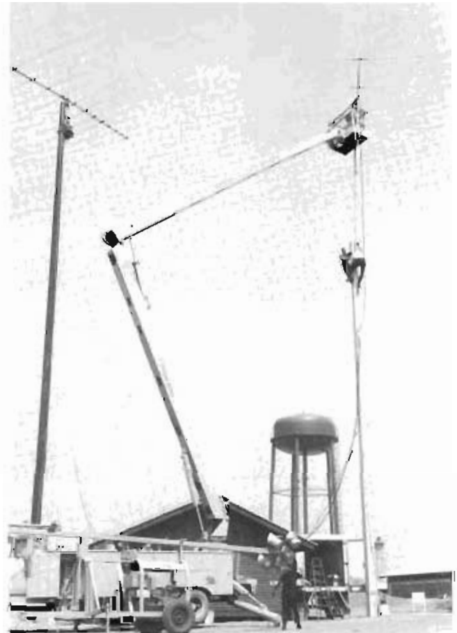
Air Force and Thai personnel use a "cherry picker" to install an antenna at the Military Affiliate Radio Station at Nakhon Phanom AB, Thailand.
