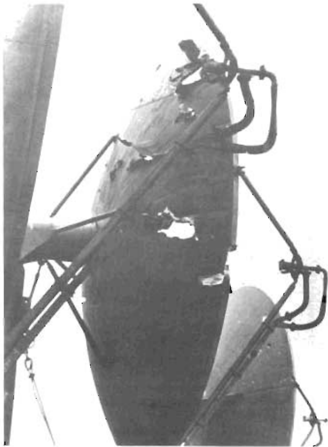
Mortar attacks damaged this signal site at Vung Chua, South Vietnam, in 1968.
