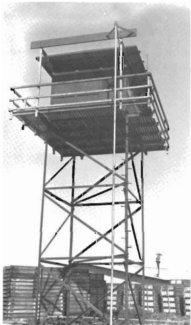
In some cases, AACS relied on prefabricated control towers to shorten the time required by a detachment to become operational. Such a tower could be shipped by air and could be erected in 100 man-hours. These photographs show the tower ready for shipment and after being assembled.
