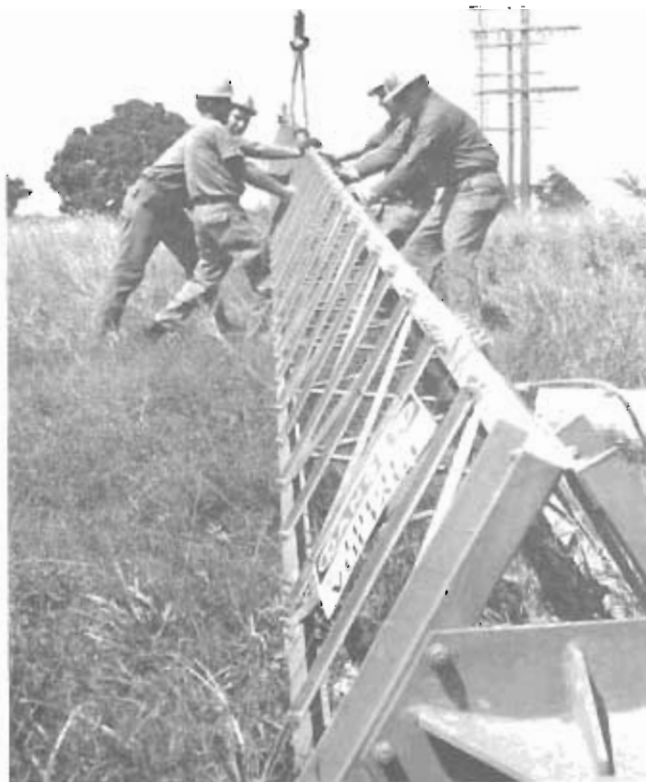
Members of the 217th Electronics Installation Squadron of the Illinois Air National Guard put some muscle into placing an antenna tower at Antigua AS, British West Indies, to aid the AFCS support of NASA projects.
