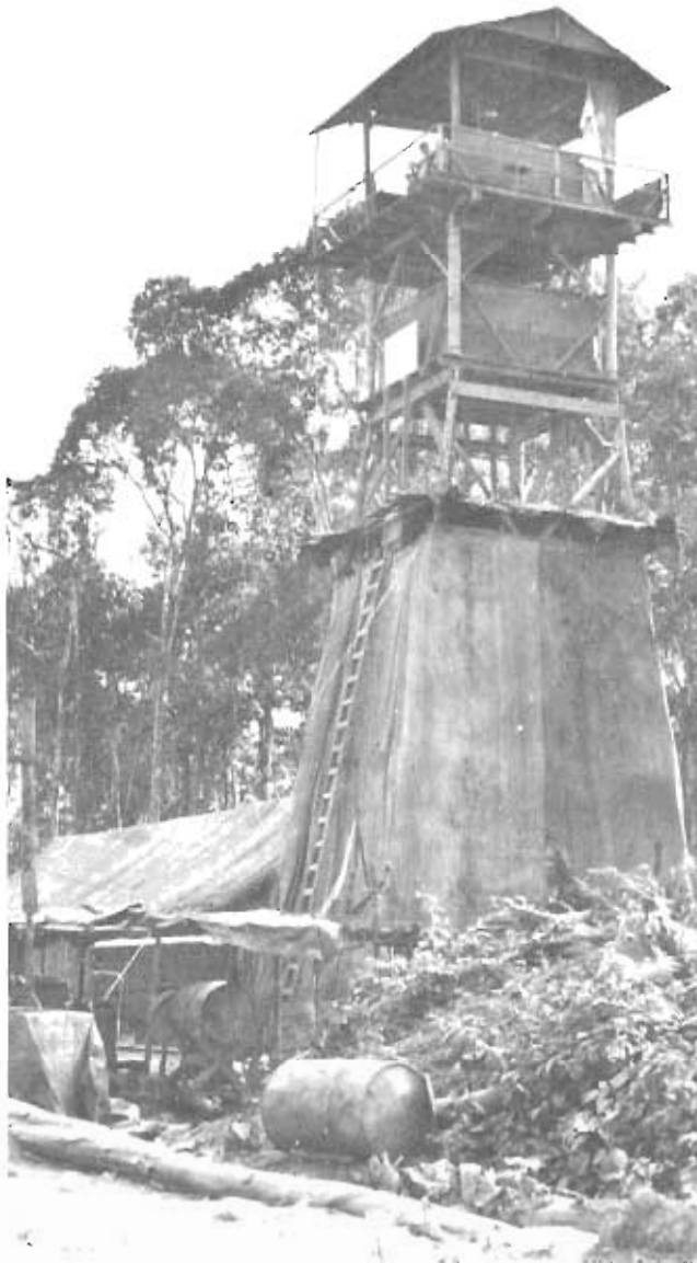
Heavy jungle had to be cleared and sites leveled before this tower in Burma could be built and before any airstrip could function efficiently. The tower belonged to the 4th AACS Wing.
