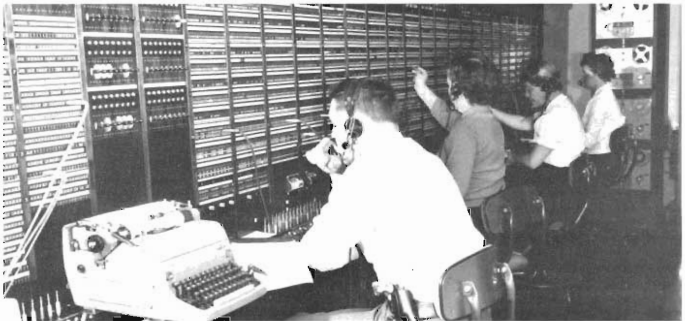
Upon its activation in 1961, AFCS assumed control of telephone systems for the Air Force. The next ten years witnessed many advancements in providing an internal telephone capability for the entire Defense Department with AFCS providing the initiative in development. Here, operators connect calls at the Washington switchboard in the USAF Communications Center at the Pentagon.
