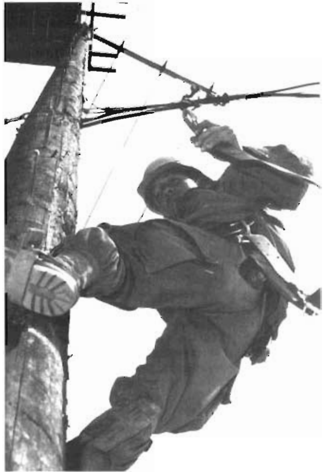
A communications technician installs an antenna for the Military Affiliate Radio System station at Pleiku AB, South Vietnam.
