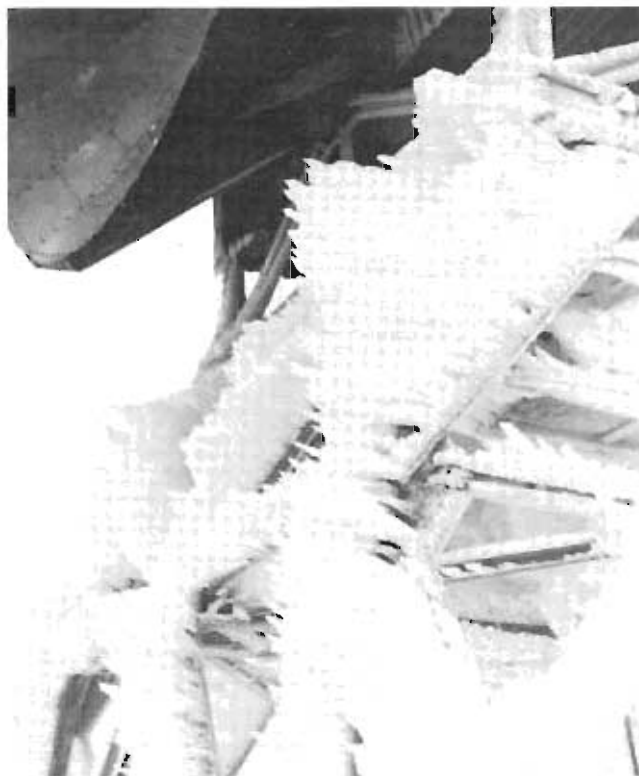
Ice and snow driven by the severe arctic winds accumulate on antenna supports at Cape Lisburne AFS, Alaska.
