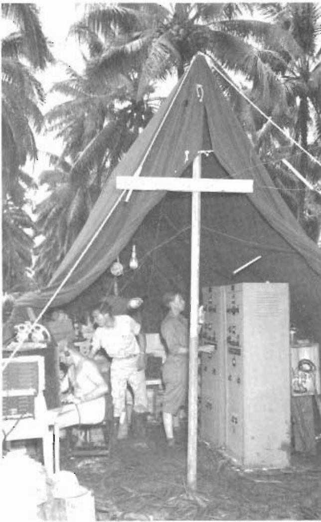
Despite ankle-deep mud, the radio station on Mission Island, in the Green Island Group, is in operation. The transmitting and receiving equipment has been set up; the generators have been started, and the first powerful signal has been sent out. March 1944.
