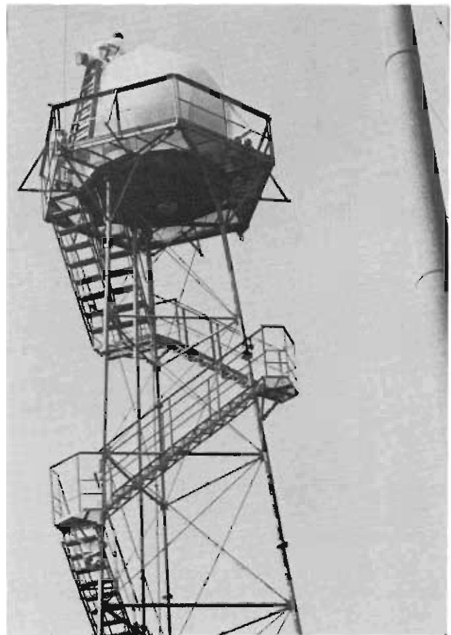
AFCC had a tone-down program to repaint some of its equipment, such as this AN/FPS-77 weather radar, to make it less visible.
