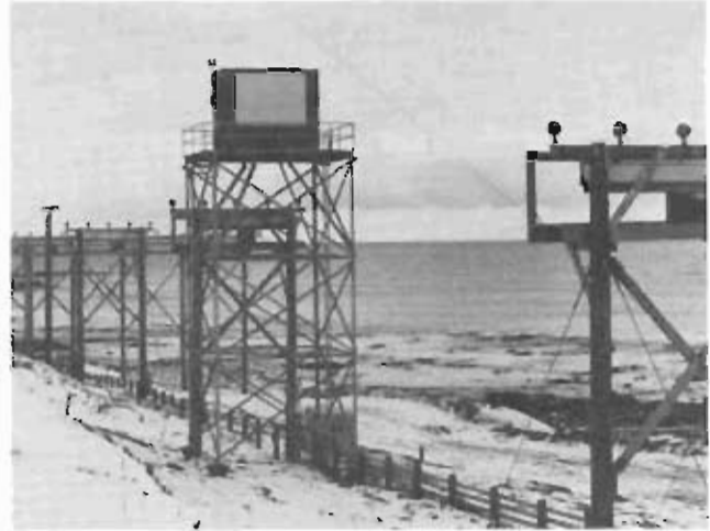
This 2-degree azimuth facility on its 30-foot tower was part of the microwave landing approach system at Shemya AFB, Alaska.
