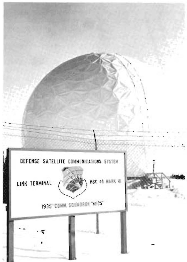
This satellite link terminal was operated by the 1935th Communications Squadron at Wildwood AS, Alaska.
