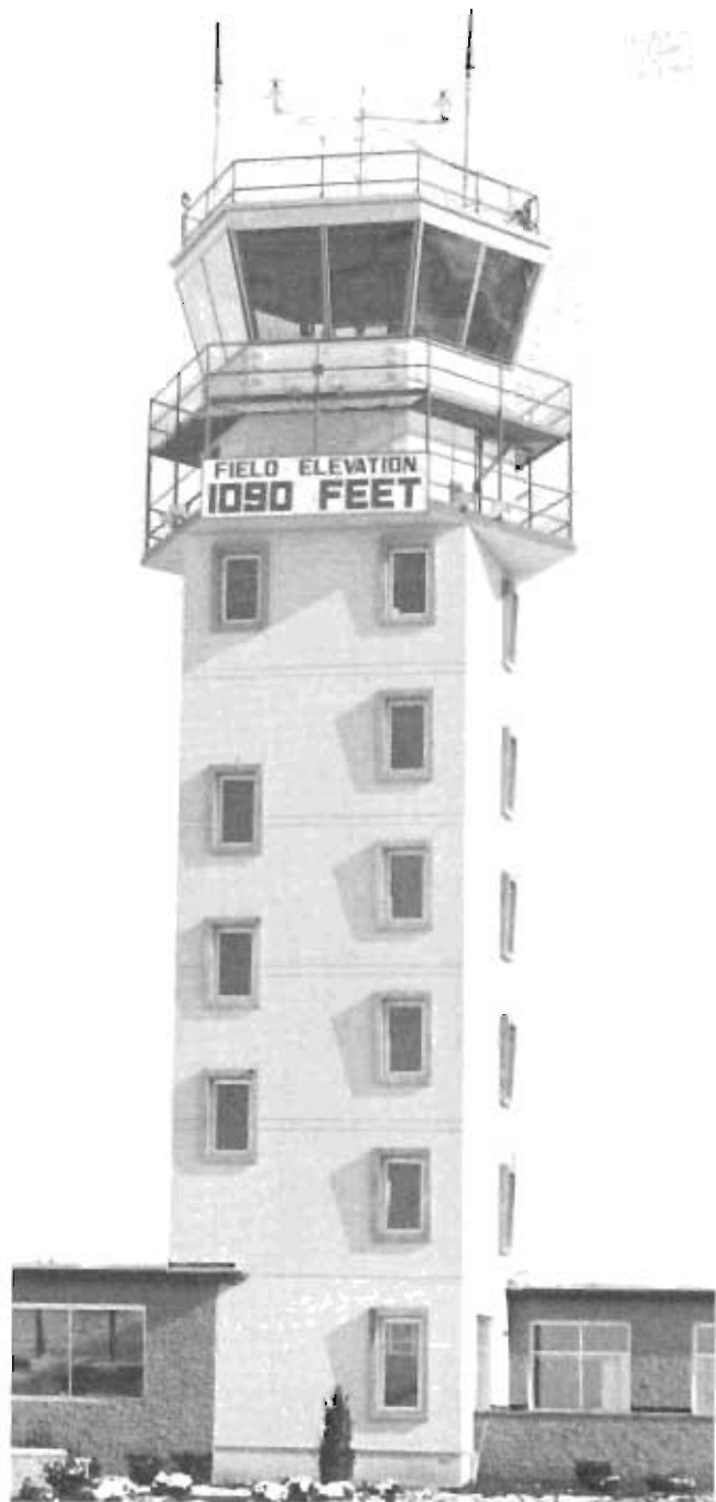
Modernized control tower and support offices at Richards-Gebaur AFB, Missouri.
