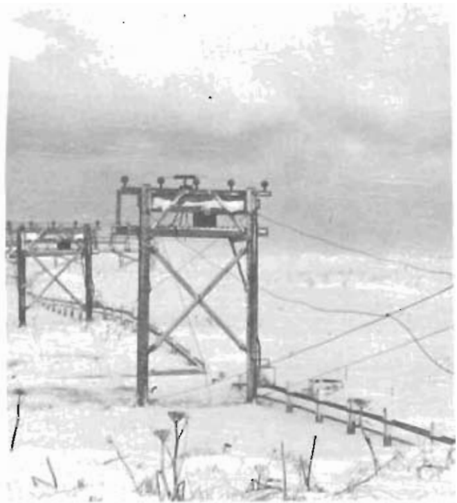
The Alaskan earthquake damaged or destroyed much of the state's communications facilities, including the air traffic control approach lights in this picture.
