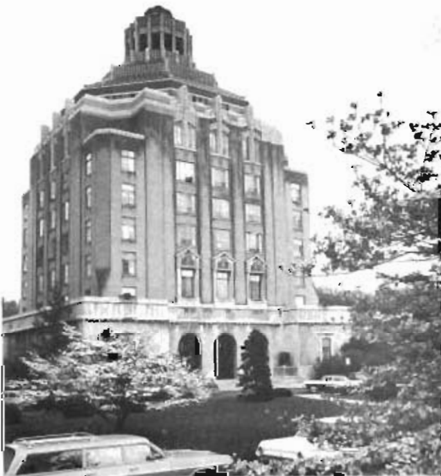
The city building of Asheville, North Carolina, served as headquarters for AACS from 3 May 1943 to 17 December 1945.
