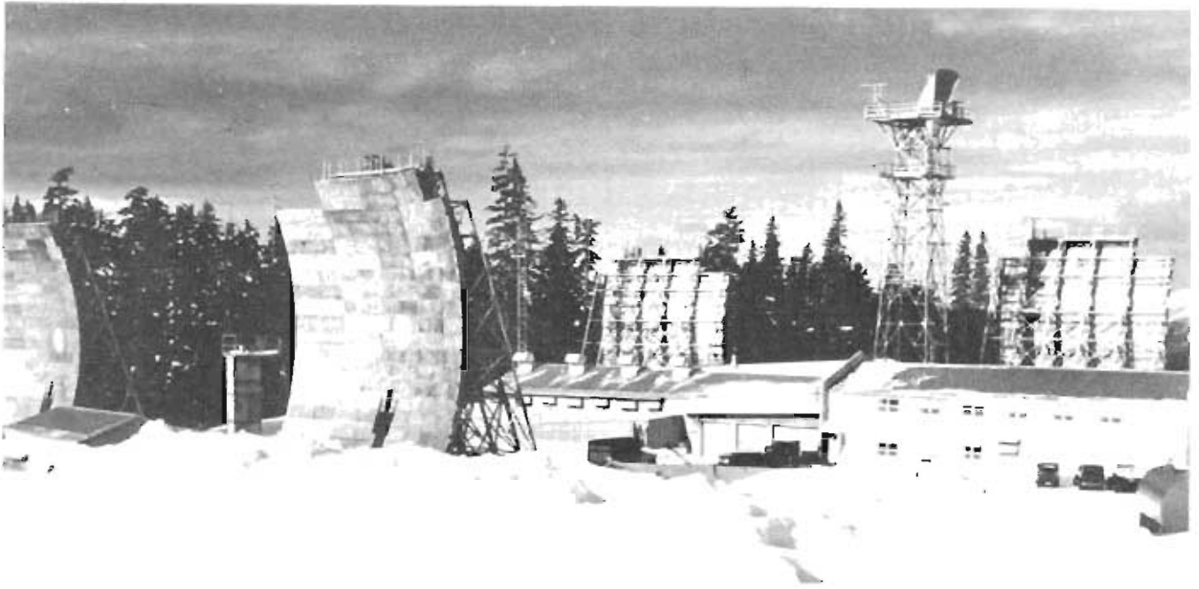
White Alice sites such as this one provided the heart of the long-haul communications system in Alaska.
