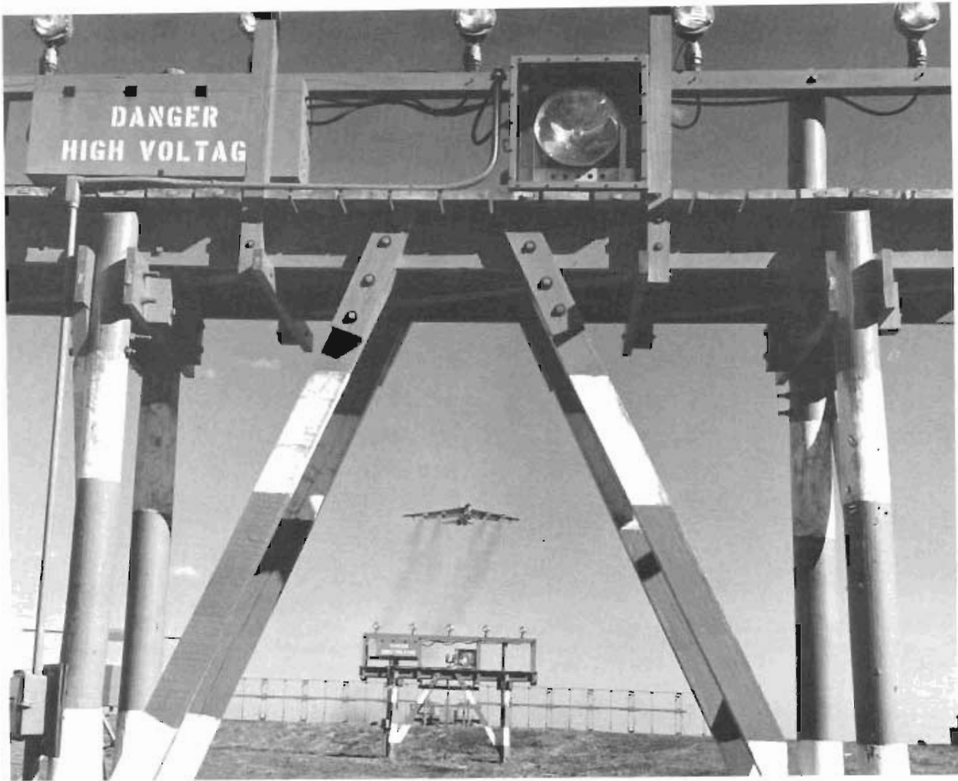
A B-52 flies over an instrument landing system which gives glide slope and azimuth for aircraft on their final approach.
