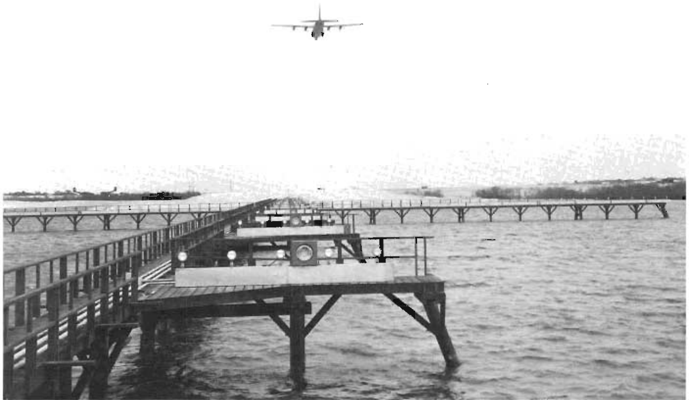
A C-130 Hercules aircraft flies over an extensive strobe-light system which points toward the landing strip at Cam Ranh Bay AB, South Vietnam. The lights are turned on by the control tower during inclement weather.
