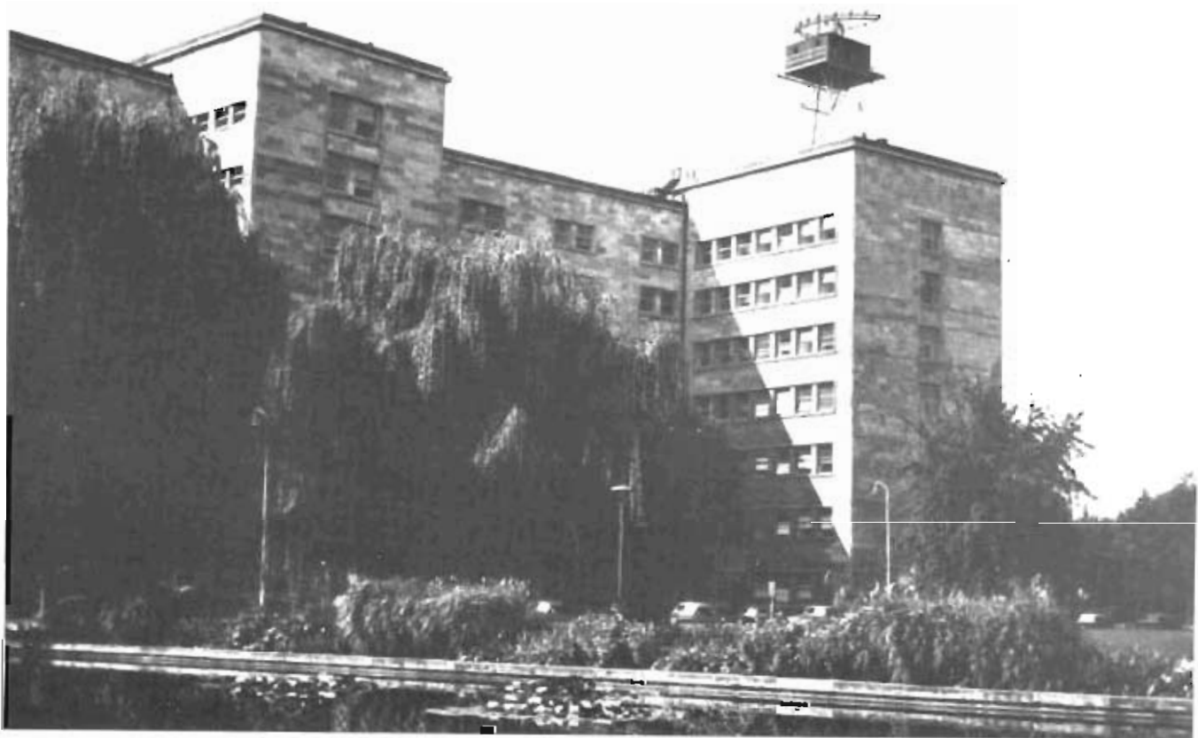
One AACS CPS-5 area control radar set was placed atop the I.G. Farben Building in Frankfurt, West Germany. The set was used in conjunction with the AACS Radar Control Center in 1950.
