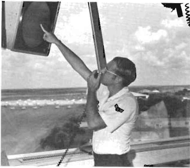
This BRITE II radar facility was added to many AFCC control towers to improve air traffic control services.
