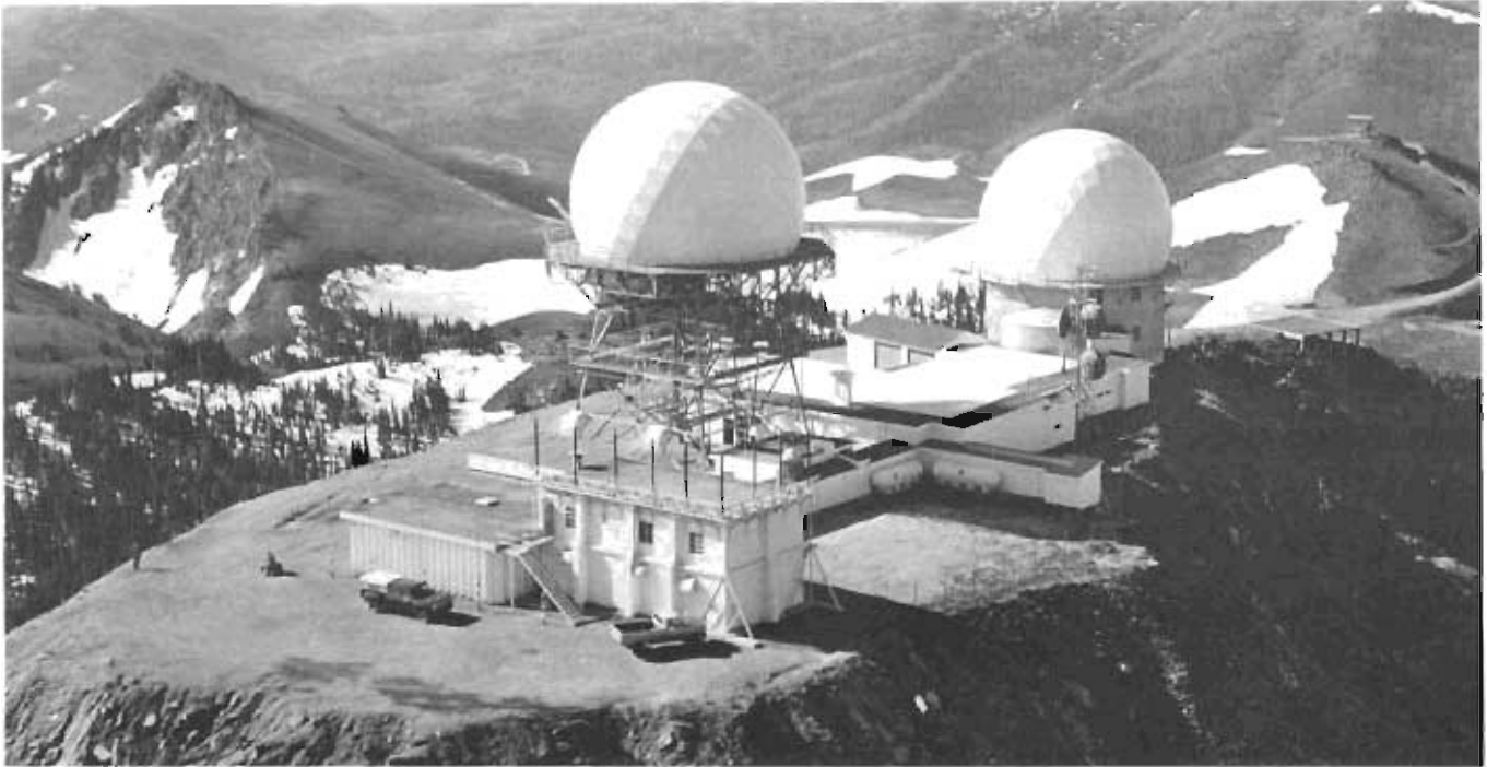
A remote radar site is perched high atop Francis Peak, Utah, operated by the 299th Communications Flight of the Air National Guard.
