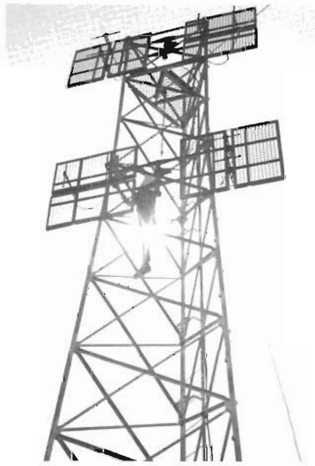
Finishing touches are completed on a new communications tower.
