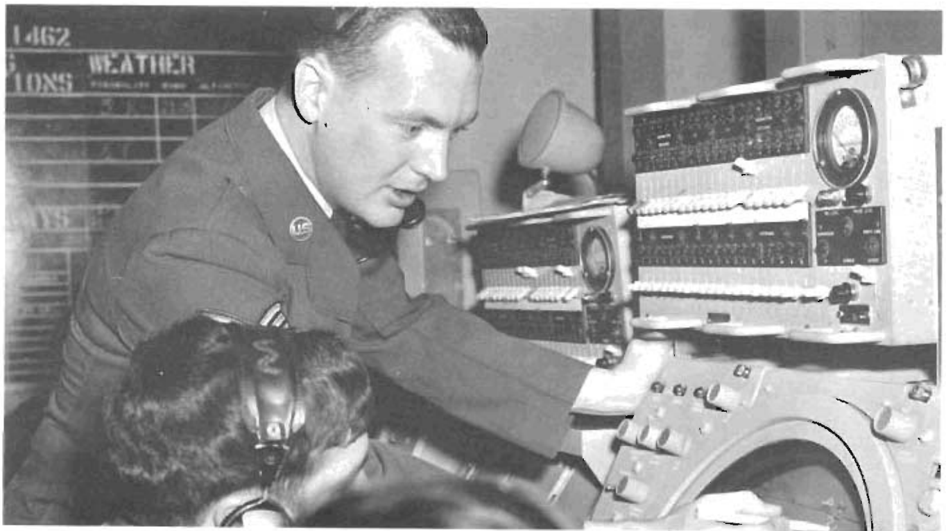
Mobile tactical air navigational facilities, such as this one at Udorn AB, Thailand, provided air traffic services to aircraft in areas that lacked fixed equipment.
