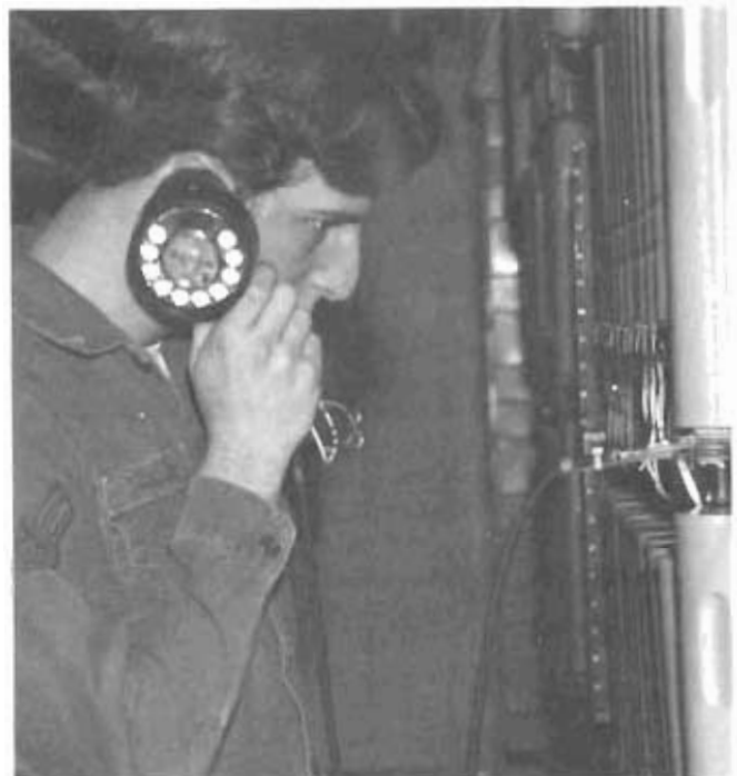
A maintenance technician with the 1974th Communications Group uses a handset to monitor a telephone line.
