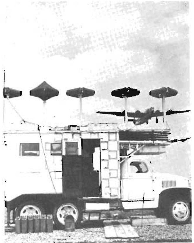
Instrument landing trucks such as this one enabled aircraft to land safely. This truck is assisting a B-24 Liberator at Smyrna, Tennessee.
