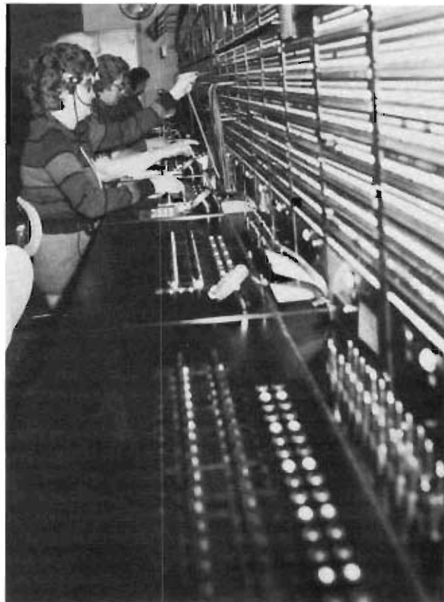
Kelly AFB, Texas, telephone operators operate the old switchboard for the last time. The next day the telephone switching system was replaced by a state-of-the-art digital switching system. This replacement was part of an AFCC program known as Scope Dial, a project to modernize base telephone systems around the world.
