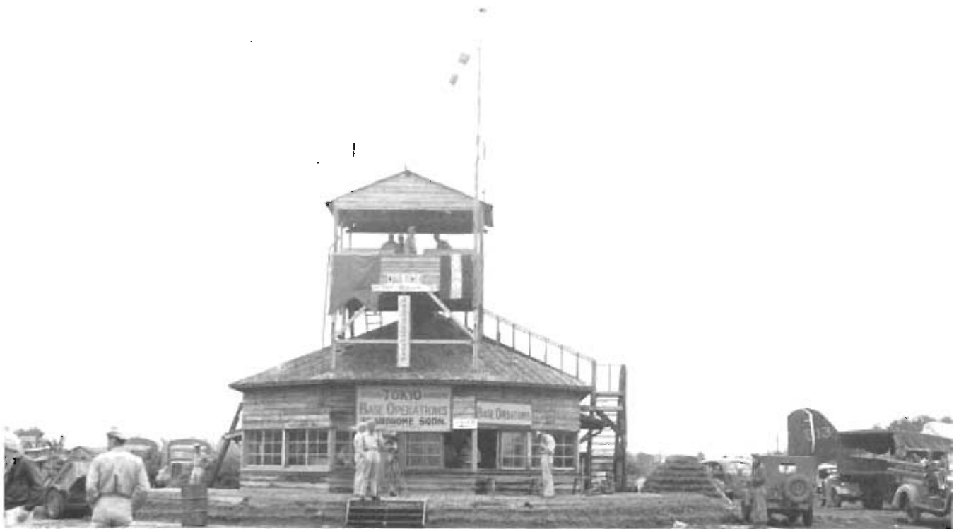
The first American control tower in Japan after the war was built at Atsugi Airfield in eight hours on 28 August 1945. On top of the base operations building was a wooden platform which the Japanese had used as a tower, but the AACS radio equipment and plans for all weather operations demanded a better structure. At the first meeting of the officers of the reconnaissance party, Col Gordon Blake, Commanding Officer of the 7th AACS Wing, voiced the desire for a tower and the engineering officers sent over a workforce of conscripted Japanese. At first, they said that it would take them through the next day to finish the job, but when they heard that lights would be provided and that the structure had to be ready by five the next morning, they promised to finish it by seven that night. When the AACS men returned from dinner, they found the tower complete with a built-in desk for the equipment and one of the Japanese sleeping on the desk, waiting for approval so that he could go home.
