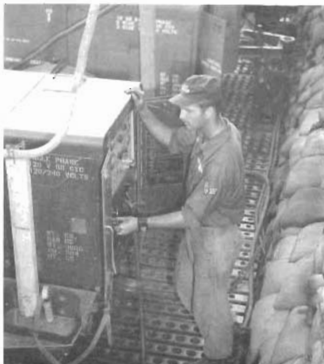
In 1965, many locations in Southeast Asia were forced to rely on revetted power units, such as these deployed to Phan Rang AB, South Vietnam.
