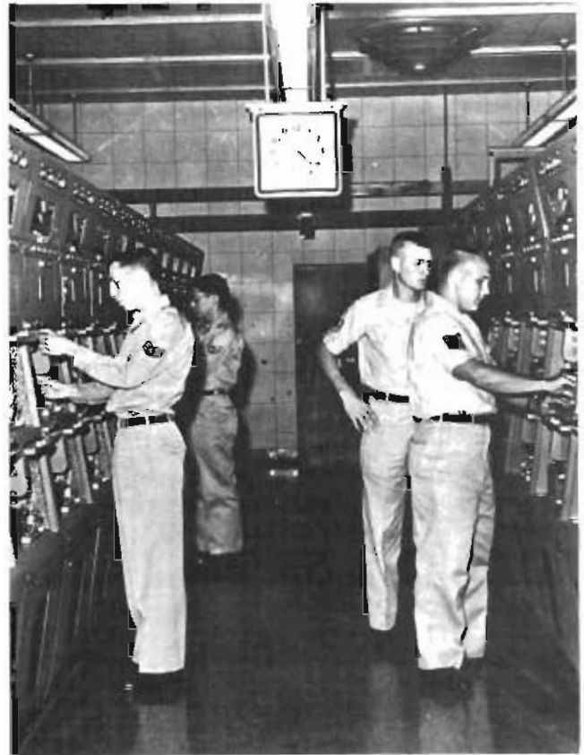
AFCS airmen check equipment in the "Plan 55" Automatic Teletype Relay at Andrews AFB, Maryland. Incoming teletype messages, received at 60 to 100 words per minute are read, automatically "switched" across the center at a rate of 200 words per minute, and sent to the addressee at the speed his equipment will receive it.
