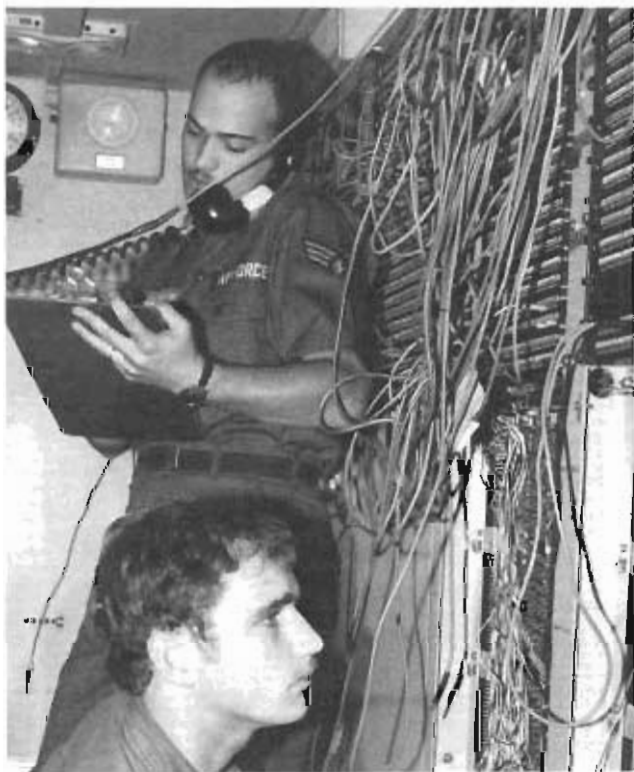
AFCS personnel from the 2d Mobile Communications Group work with a maze of patch cords and wiring in a technical control van to maintain circuit continuity between various communications facilities.
