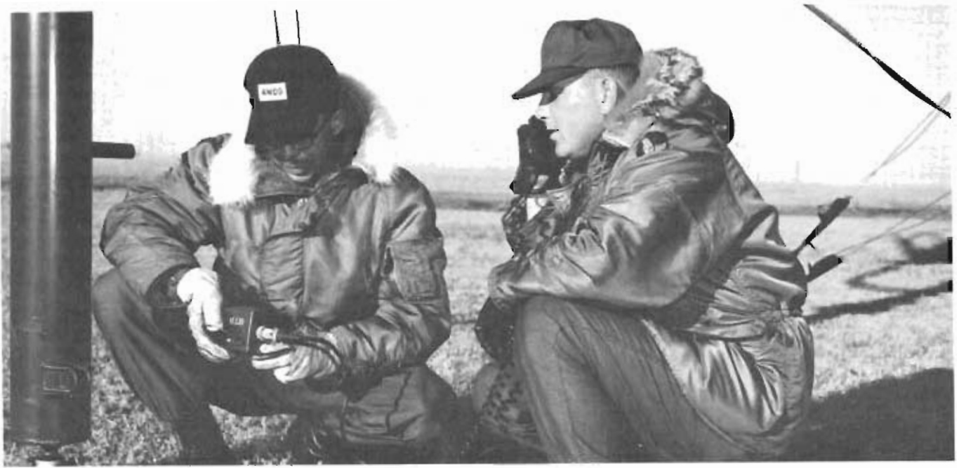
Two AFCS members check control tower equipment during a field test of the 4th Mobile Communications Group.
