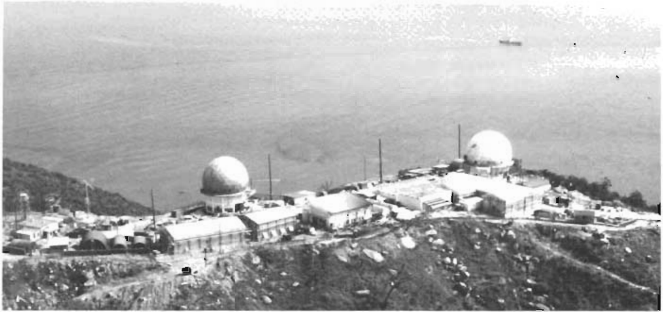
A communications site near Monkey Mountain, South Vietnam.
