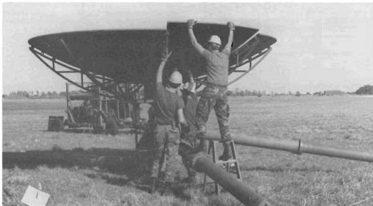
Members of the 2d Combat Communications Group's Satellite Communications Branch assemble the TSC-100 satellite dish during an operational readiness inspection in which every aspect of the unit's wartime mission was evaluated.
