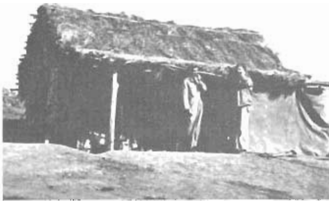
Control tower at Tontouta Field, New Caledonia, September 1942.
