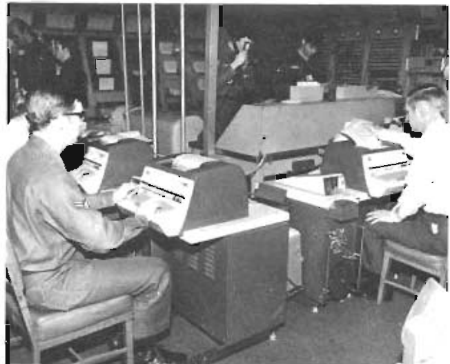
Manual technical control facilities provide a background from the automated technical control teletypewriter as installed in the technical control facility at RAF Croughton, England.
