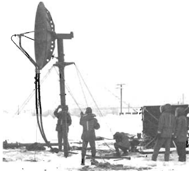
Members of the 5th Combat Communications Group install an 8-foot parabolic antenna at Eielson AFB, Alaska. The antenna is part of a system to provide communications and air traffic control services during mobilization.
