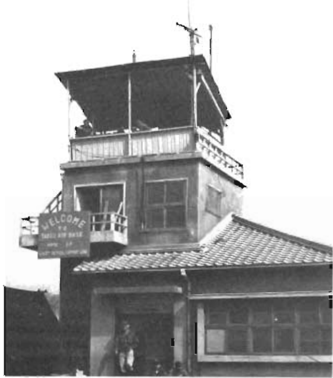
Typical of the ingenuity of the U.S. Air Force in Korea is the addition of the perch atop an old Korean building at Taegu, in order to provide an "open air" control tower for operations of our fighter strips located here, October 1950.
