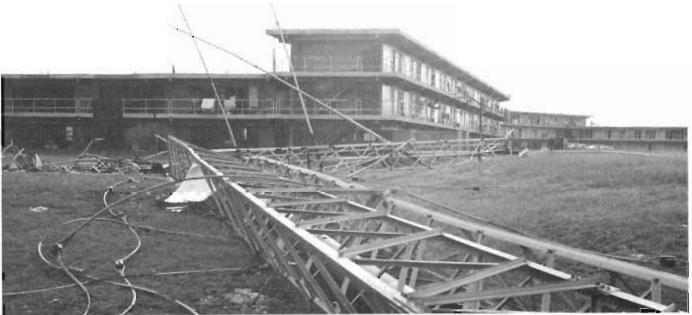
A communications antenna that supported the Strategic Air Command GIANT TALK program was felled by typhoon Pamela on Guam in 1976.
