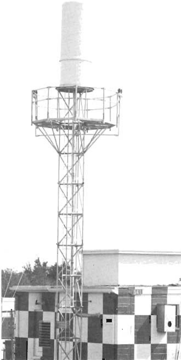
Tactical Air Navigation equipment and generator support buildings. This equipment provides aircraft omnidirectional azimuth, identification, and distance information.
