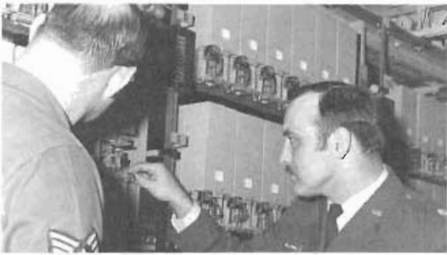
The base communications-electronics officer from the 2167th Communications Squadron at RAF Chicksands, England, checks the frame room in the Base Consolidated Switchboard, which handles commercial and AUTOVON lines.
