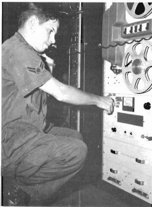
An AFCS airman assigned to the 1880th Communications Squadron makes a daily equipment quality check of a recorder used in the Binh Thuy AB, Vietnam, Air Traffic Regulation Center. The equipment is used to record all voice communications between aircraft and the center.
