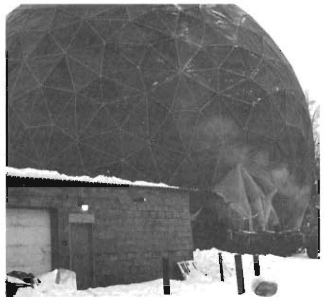
The radar dome to house the AN/MS-46 satellite communications terminal at Elmendorf AFB, Alaska, was constructed during 1974.
