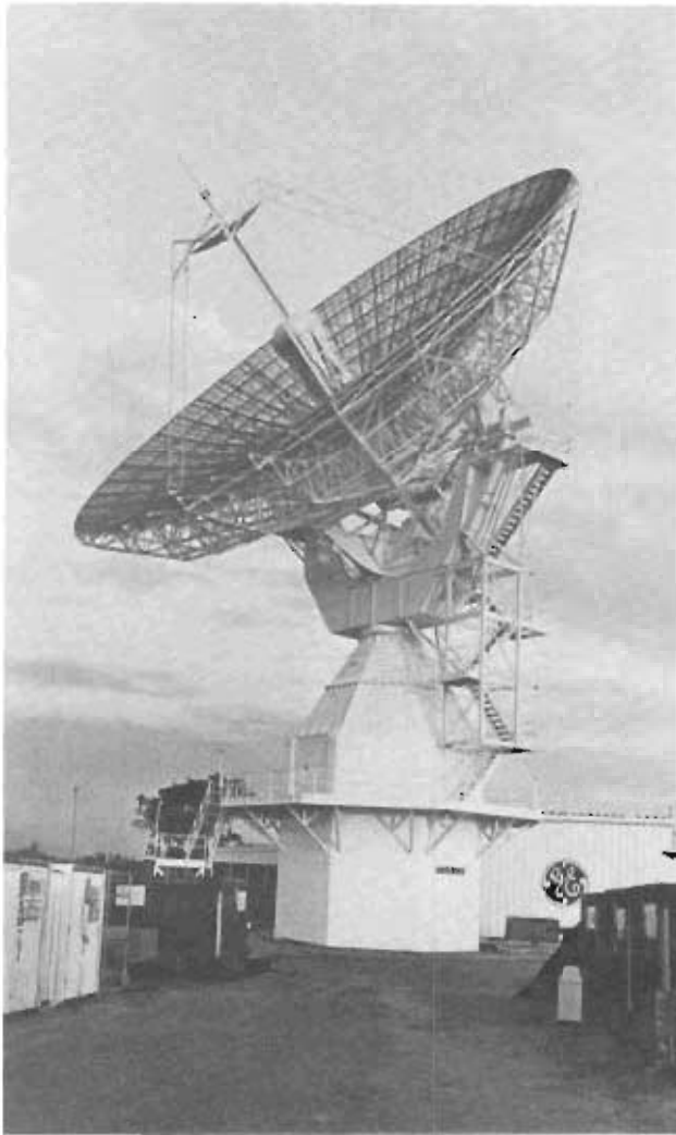
"Giant Sapphire" is an 85-foot AN/GPS-10 radar used to detect and track new foreign launches and orbiting satellites from its location at San Miguel Naval Communications Station, Philippines. Members of Space Communications Division, Detachment 2, maintain the communications-electronics equipment necessary to transmit information between San Miguel and North American Aerospace Defense Command's Cheyenne Mountain Space Surveillance Center in Colorado.
