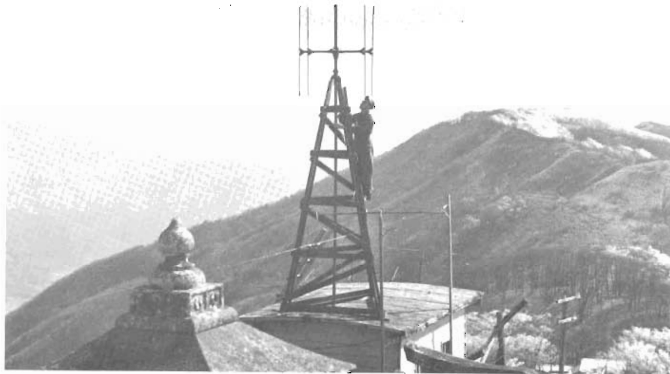
Directional finding antennas, such as this one in Japan, were the lifeline for aircraft flying between Japan and Korea. These systems, operating 24 hours a day, provided radio navigational aid to hundreds of aircraft daily.
