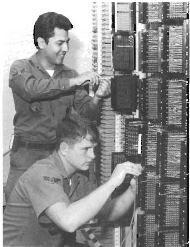
A1C Christopher Finch and A1C Larry Gusman of the 392d Communications Group telephone maintenance work center, Vandenberg AFB, California, troubleshoot a key telephone system.
