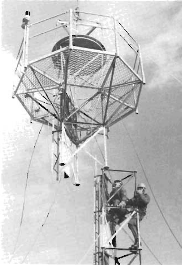
SrA James Fink and SrA Andrew Hyde prepare to mount the crow's nest for the TACAN antenna at Grand Forks AFB, North Dakota.
