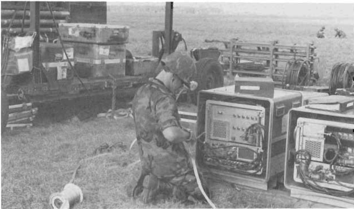
A 2d Combat Communications Group member hooks cable to electronic equipment during the build-up phase of an operational readiness inspection.
