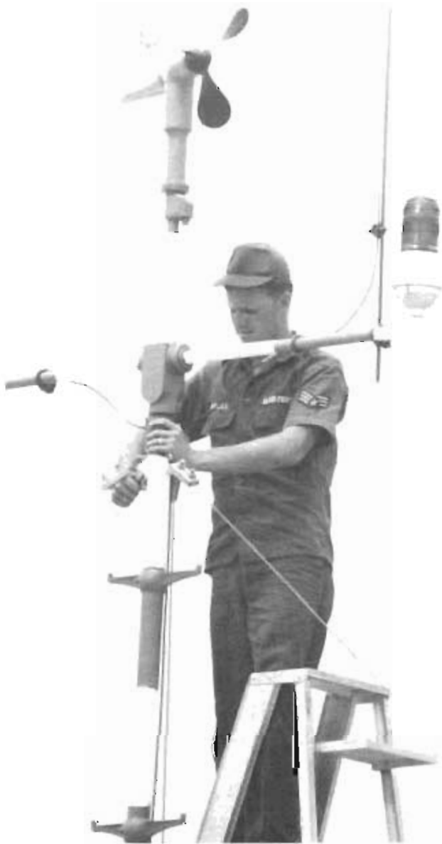
Demands for increased weather support prompted the installation of fixed meteorological equipment throughout the combat area. This wind speed and direction set provided crucial data to Air Force personnel responsible for forecasting weather.
