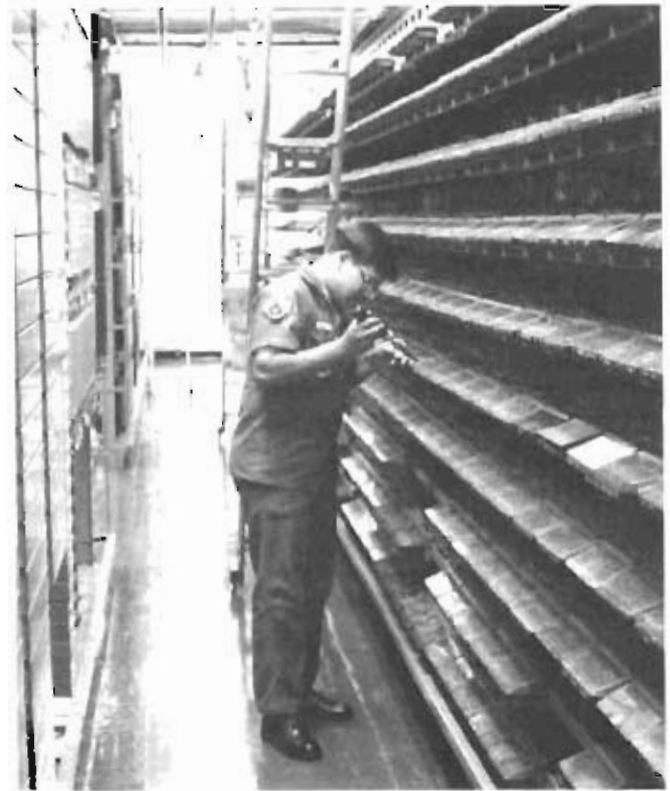
An AFCS technician performs preventive maintenance on the Norton AFB, California, telephone switchboard mainframe.
