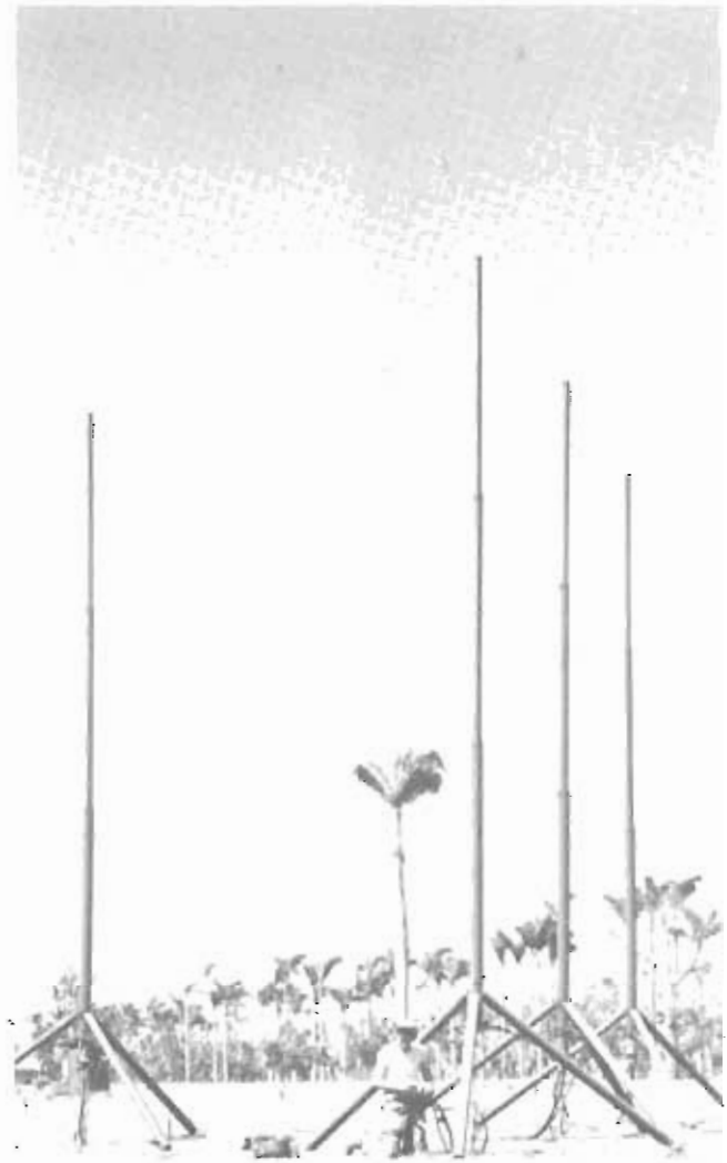
Pictured here is one of AACCS's mobile range stations used to broadcast radio beams, which served as highways in the air for Army Air Force planes. These stations enabled the armadas of Boeing B-29 bombers striking Japan to return to bases on pinpoint islands in the vast Pacific in instrument weather.
