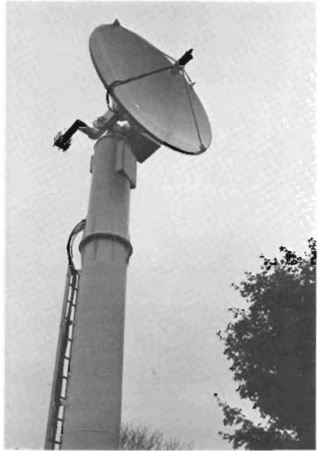
The 8-foot dish of the Search and Rescue Satellite-Aided Tracking System antenna at Scott AFB, Illinois, homes on a low angle satellite.
