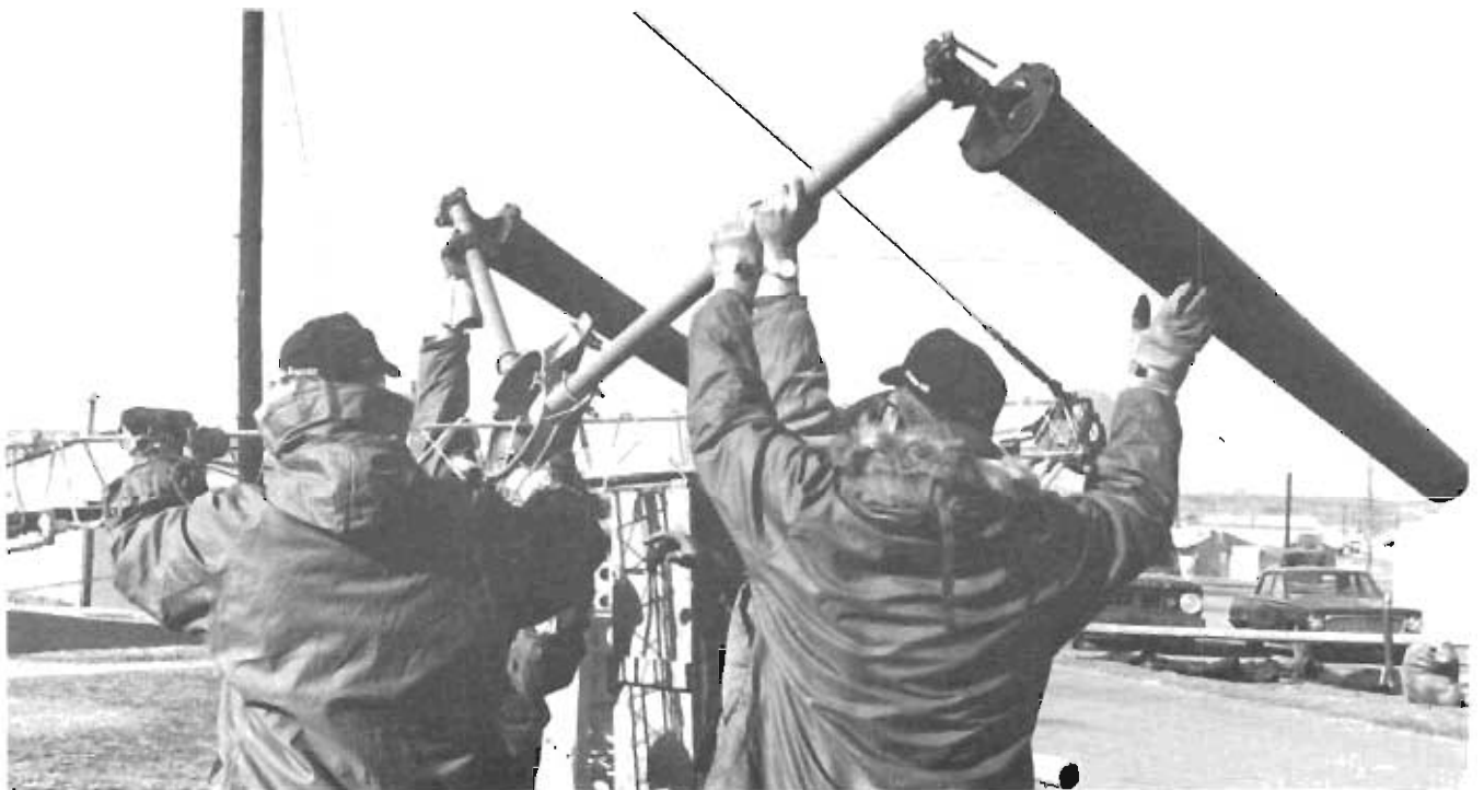
Antenna maintenance men of the 1st Mobile Communications Group add radiation domes to a 60-foot tower to provide ultra high frequency communications from airborne aircraft to the command center.
