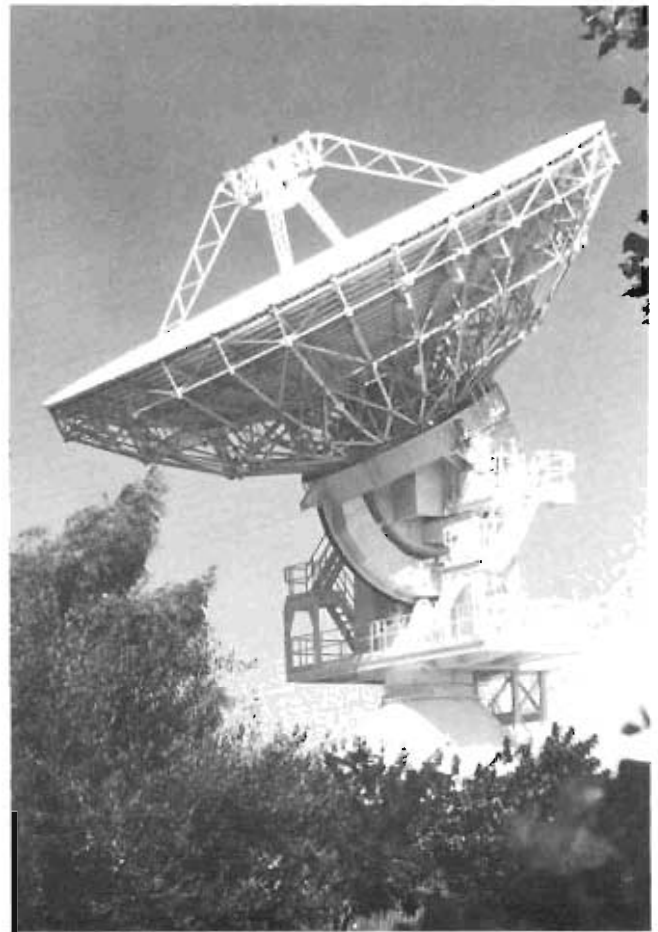
A satellite station operated by the Strategic Communications Area at Offutt AFB, Nebraska.
