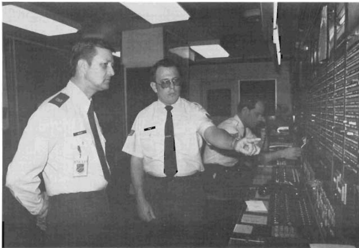
Washington D.C. tactical switchboard
