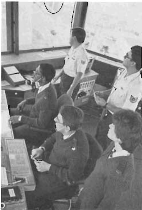
Part of AFCC's control tower modernization program included remodeling the tower cab. Members of the 1883d Communications Squadron at Beale AFB, California, gained more floor space with the new wraparound-type console.
