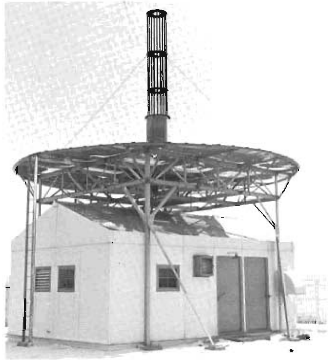
This AN/FRN-12A very high frequency omnidirectional range (VOR) provided an infinite number of radial courses, thereby permitting great flexibility in the establishment of routes.
