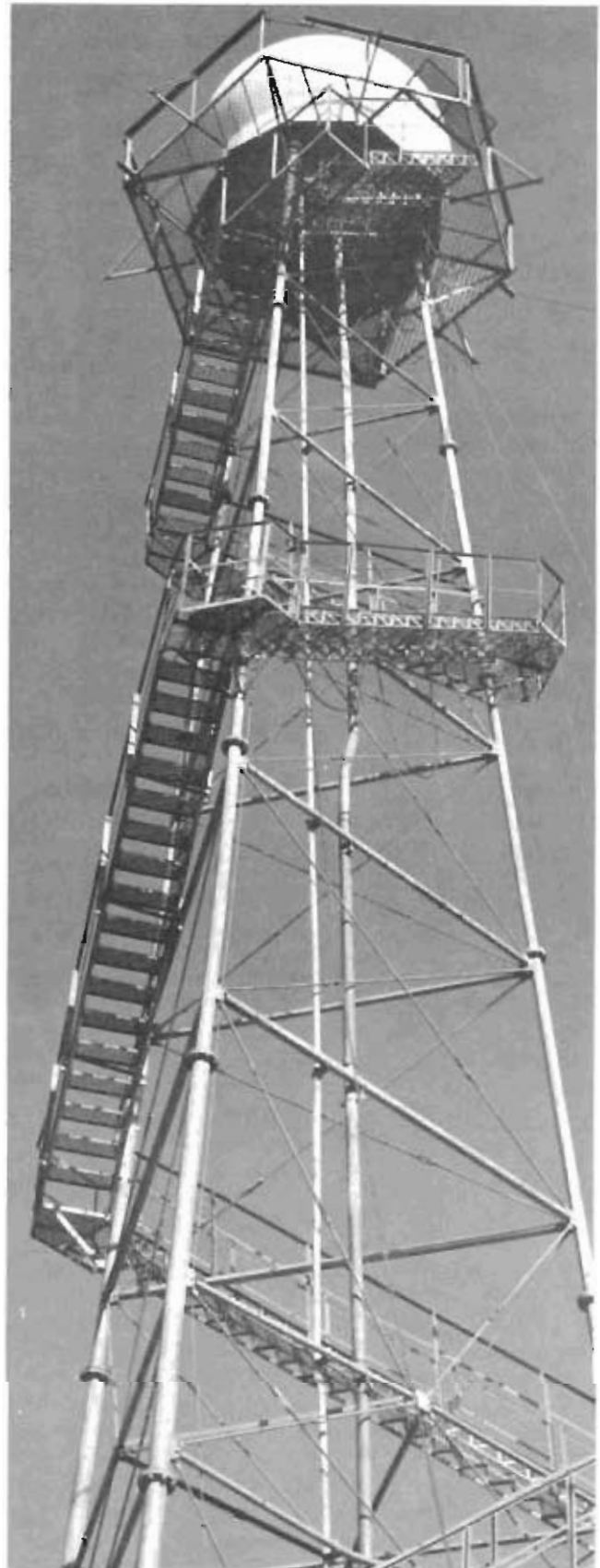
This storm-detection radar, an AN/FPS-77, was part of the Air Force weather network, operated by AFCS.
