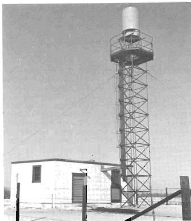
This facility is a tactical air navigation (TACAN) system.
