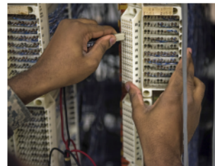
A1C Bashir Auld, 633rd CS voice systems technician, verifies phone numbers on the landlines that run across the base. They record what building and room each number goes to for when someone calls 9-1-1.
