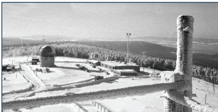
Rhein Control Tech Site on Erbeskopf Mountain with the GPS 4 radar.
