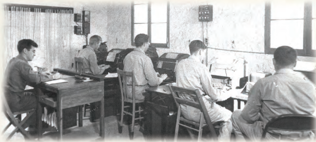
Perforated tapes for transmission hang on the left side of the teletype room as members of the 19th Army Airways Communications System Squadron use model 30 and 36 teletypes to send communications.
