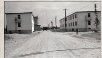
North barracks, left. Right, squadron mailroom and barracks
